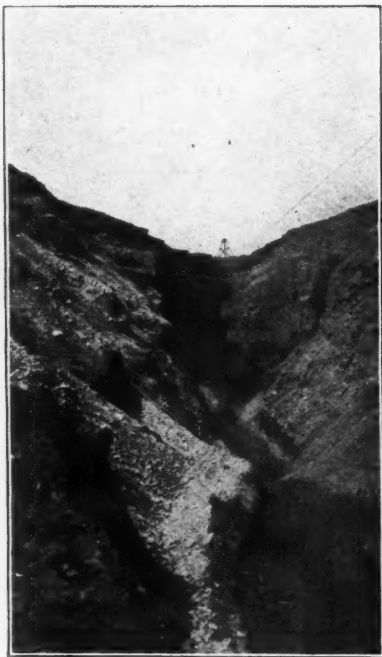
Dragline Working in Cut
